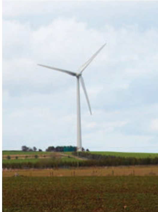
Figure 3: Two identical Enercon E-70 turbines, operated by Ecotricity, are shown. The one at Shooters Bottom in Somerset (right), is generating 5,700,000 kWh a year. The other one, beside the M4 at Green Park near Reading, (left) produces just 3,500,000 kWh. The difference is accounted for by the wind energy dissipated through friction and turbulence as a result of the surrounding buildings and trees.
