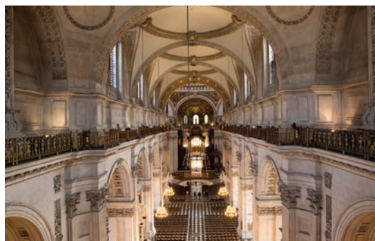
Figure 5: The refurbished heating system in St Paul's Cathedral required controls that are able to account for the building thermal inertia
