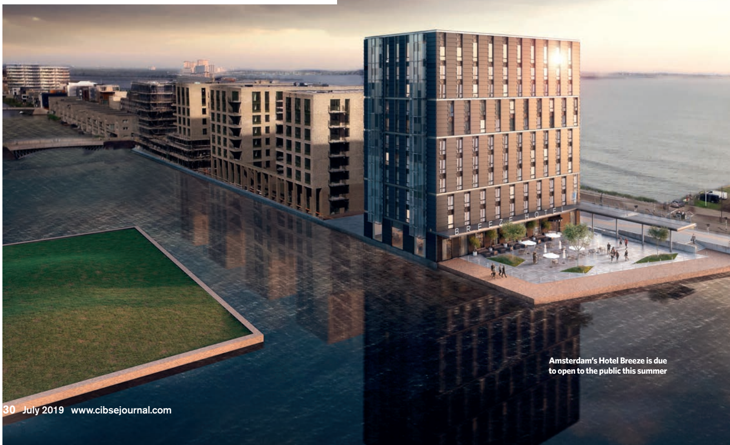
The airflow rate of the Breeze Hotel is 25.000m 3 ·h -1
