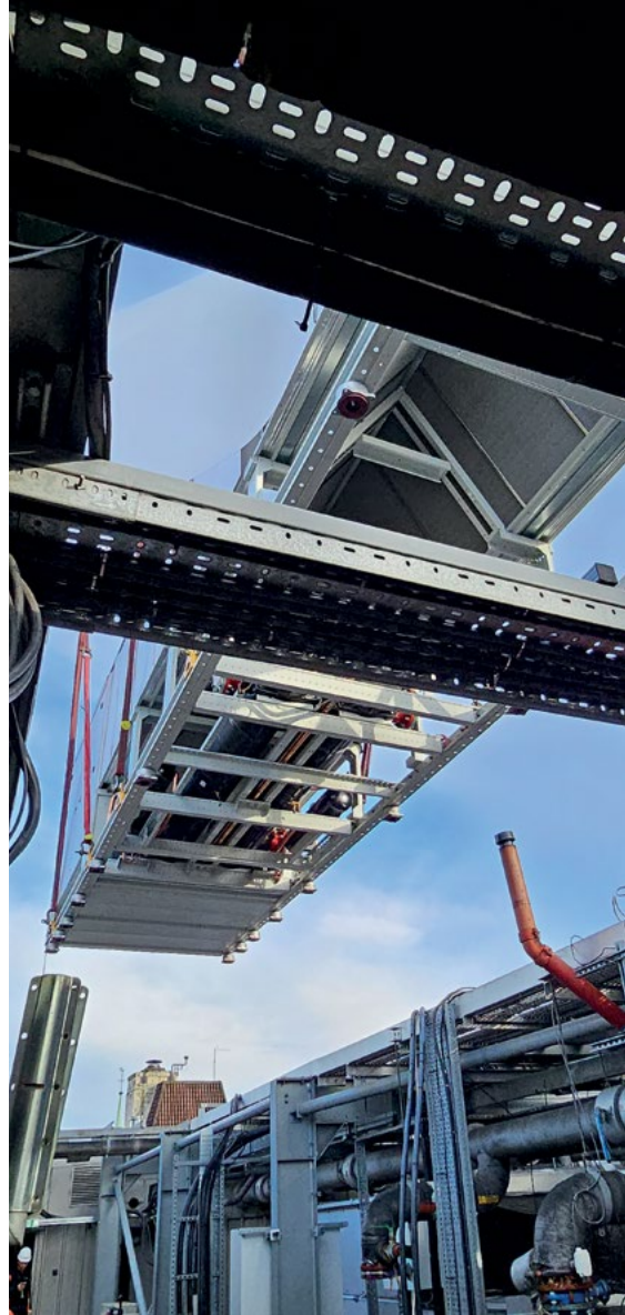
» A heat pump being craned into position
