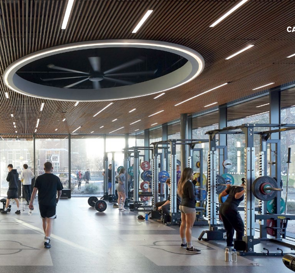
Left: One of the striking giant fans set into the ceiling in the gym. The fans have been designed to generate air movement to reduce the need to drive down the fitness suite air temperature
