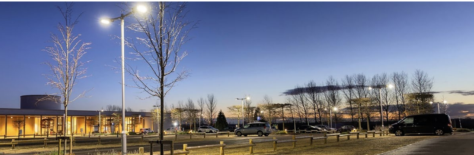
Figure 2: The parking area and pedestrian approach to the Remembrance Centre at the National Memorial Arboretum in the UK is designed to provide an environment that maintains the dignity of the location and suitable illumination for awareness of others, reinforcing a perception of safety (Source: Tamlite)
