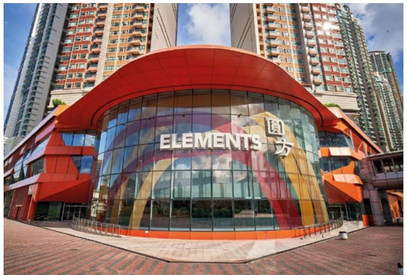
Big-data analytics cut annual energy use by 9% at the Elements MTR shopping mall
